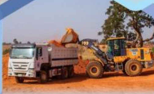
Construction of the 36km World Bank sponsored Access Road projects (RAAMP) in Plateau state
